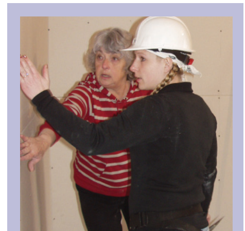
Arlene Eastman and Sarah Johnson check the nails on the drywall during the WB work day at the LaConner home on Saturday, March 1.
